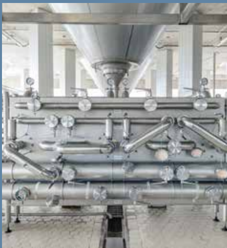
A CIP system with eleven different tanks provides automatic cleaning of the entire cold end.
